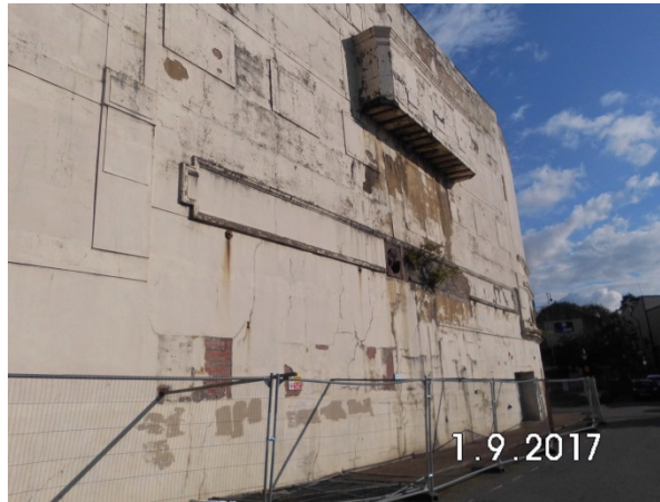
Side of theatre on Cow Lane
