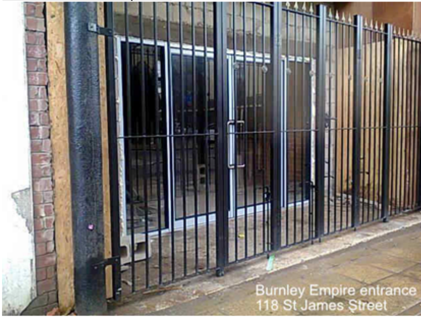
New installed shopfront
